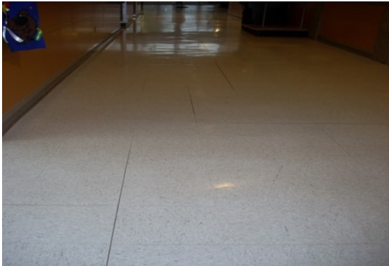
Gapped VCT from subfloor movement
