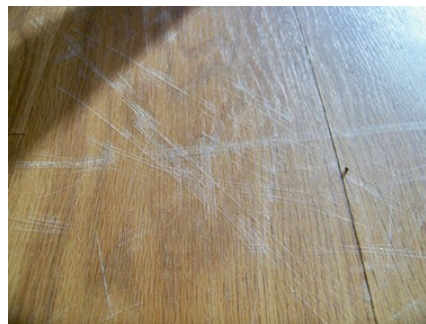
Scratches from dragging fixtures across the flooring
